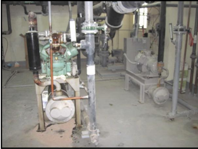
un-finished mechanical room
