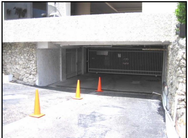
parking garage entrance
