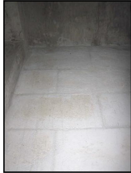
CBS wall construction, poured concrete floor & roof decks
