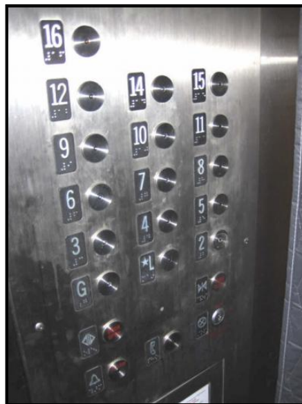
16 stop elevator panel
