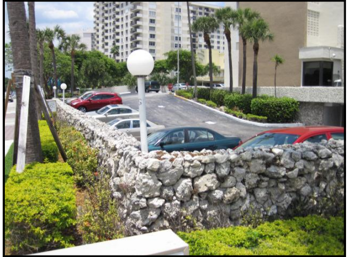
site lighting / wall
