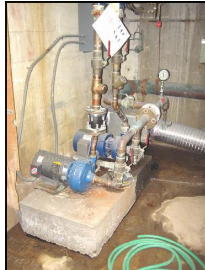
domestic water pumps
