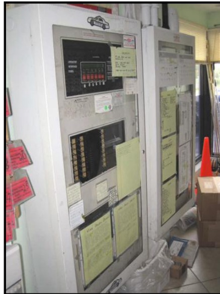
master fire alarm panel (updated 2015)
