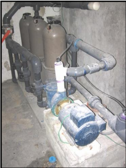
pool equipment (in garage)
