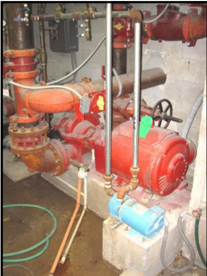
water booster / fire pump
