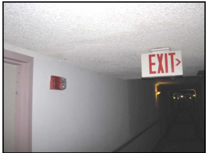
fire alarm siren/strobe, lit emergency exit sign
